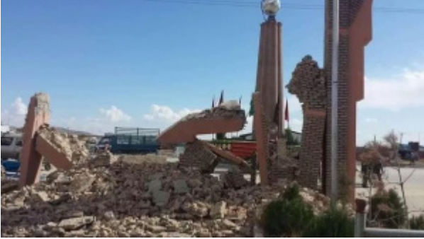
Damaged entrance of Ghazni province (Photo: courtesy Twitter)
